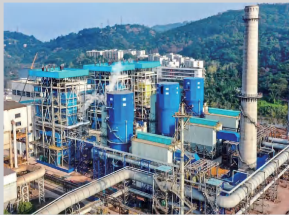
Chongqing Iron & Steel's Self-generating Energy Equipment
